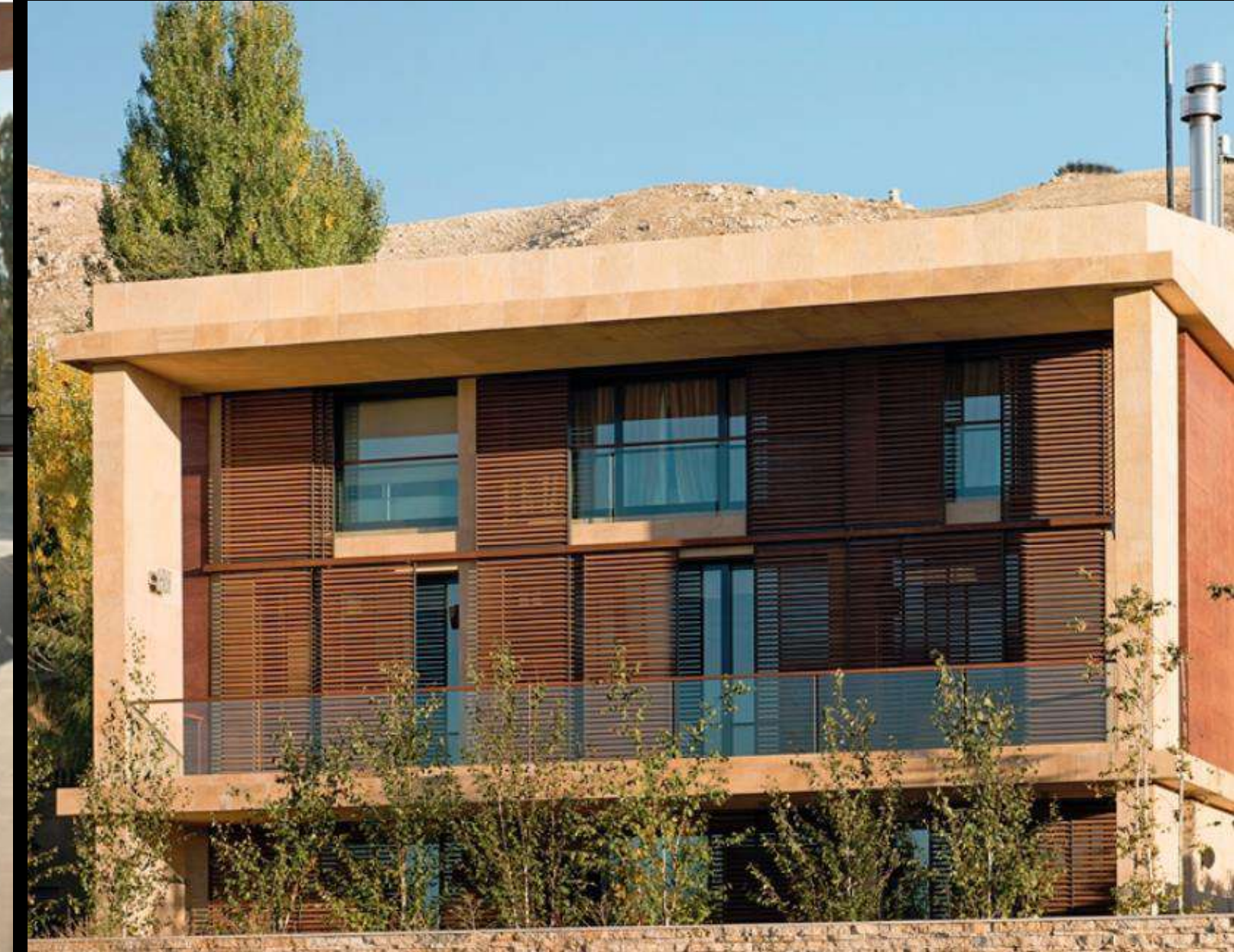
SLIDING SHUTTERS - RACHID KARAM ARCHITECTS - MOUAWAD VILLA - FAQRA - LEBANON
